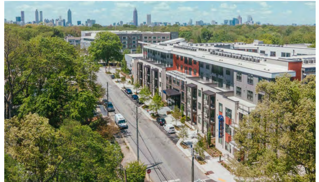
High-Density Transit-Oriented Workforce Housing | Atlanta, GA Atlanta’s public land disposition guidelines which include zoning relief for project modifications, and higher density uses and reduced parking requirements, helped the Metropolitan Atlanta Rapid Transit Authority recruit developers for station-area transit-oriented development contracts that include workforce units.
